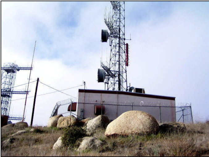
Photograph 3: View toward Box Springs candidate location, facing south.
